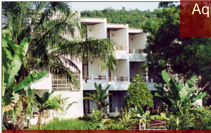
Chumphon Cabana, Resort (3 storey), Thailand (1998)
