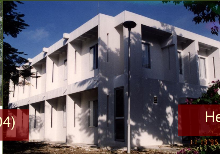
Aquaculture Outreach Office Building, Thailand (1994)
