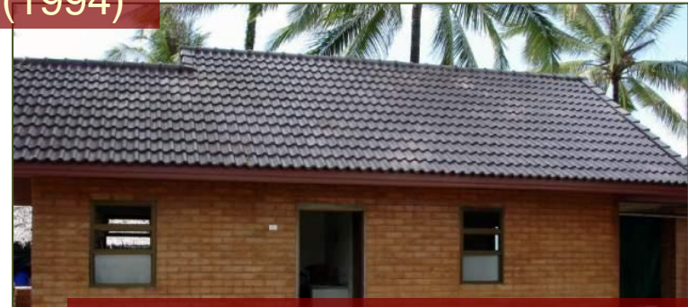
Khao Lak Resort (8 buildings), Thailand (2005)
