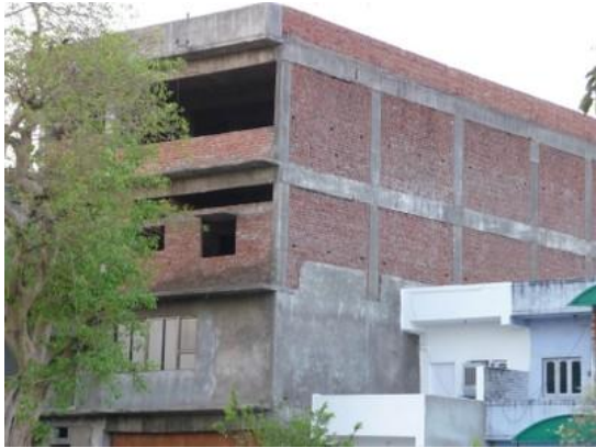
Concrete frame structure building
